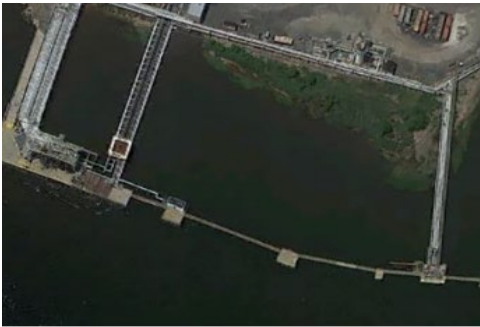
River Maintenance Dredging, NY
