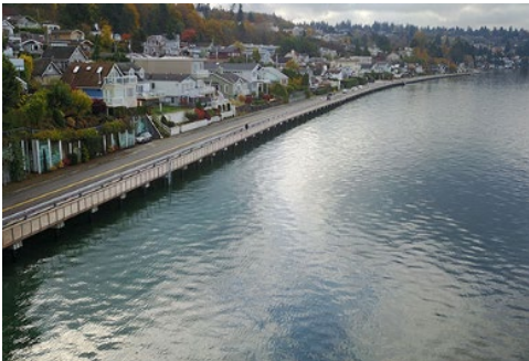
Redondo Boardwalk Repair, WA
