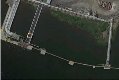
River Maintenance Dredging, NY
