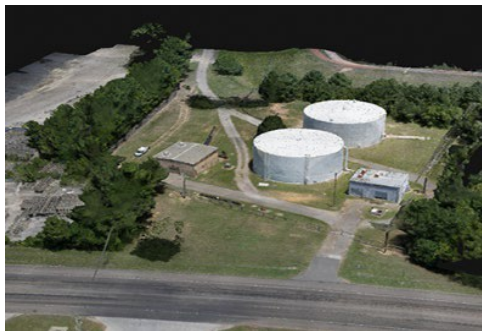
Kilgore Surface Water Plant, TX
