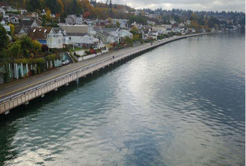
Redondo Boardwalk Repair, WA
