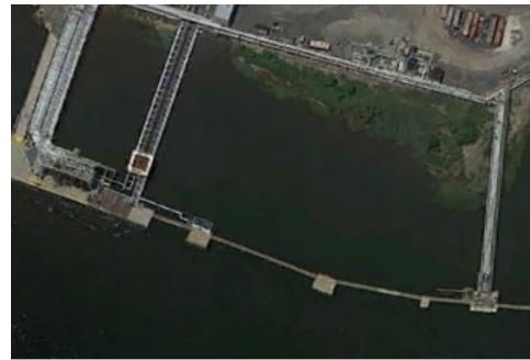
River Maintenance Dredging, NY
