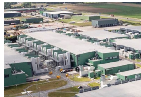
Mission Critical BYO Power
