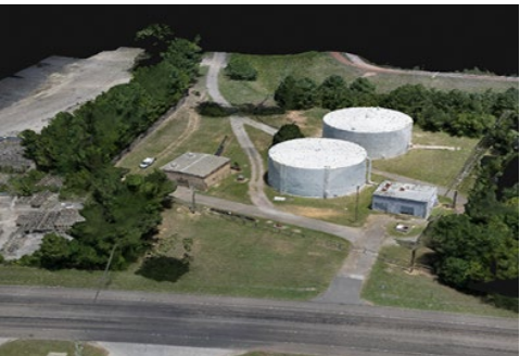
Kilgore Surface Water Plant, TX
