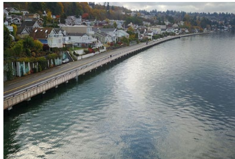
Redondo Boardwalk Repair, WA
